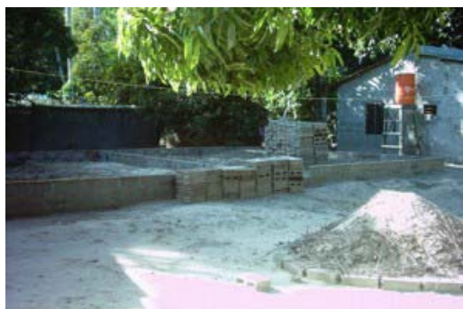
2 New Classrooms are being built, as God supplies
